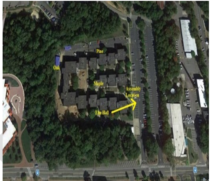
Elm Hall - Site Photo
